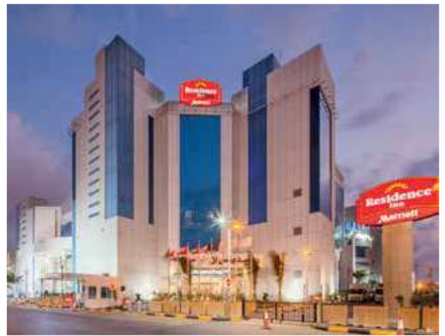
Al Rashid Mall & Courtyard - Retail & Hospitality Jazan, KSA
